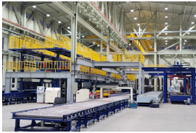
Rebar processing plant of Robocon Technologies Corp., South Korea
